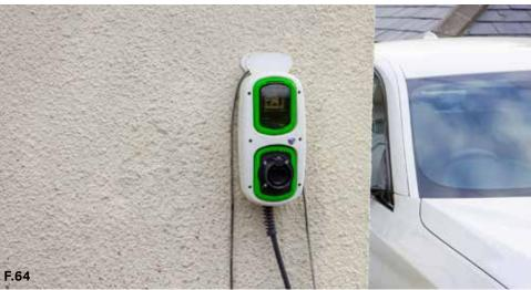
**Figure 64:** Electric charging points should be located discretely, where possible avoiding building façades visible from the road or public pathways to retain the character of the building.
