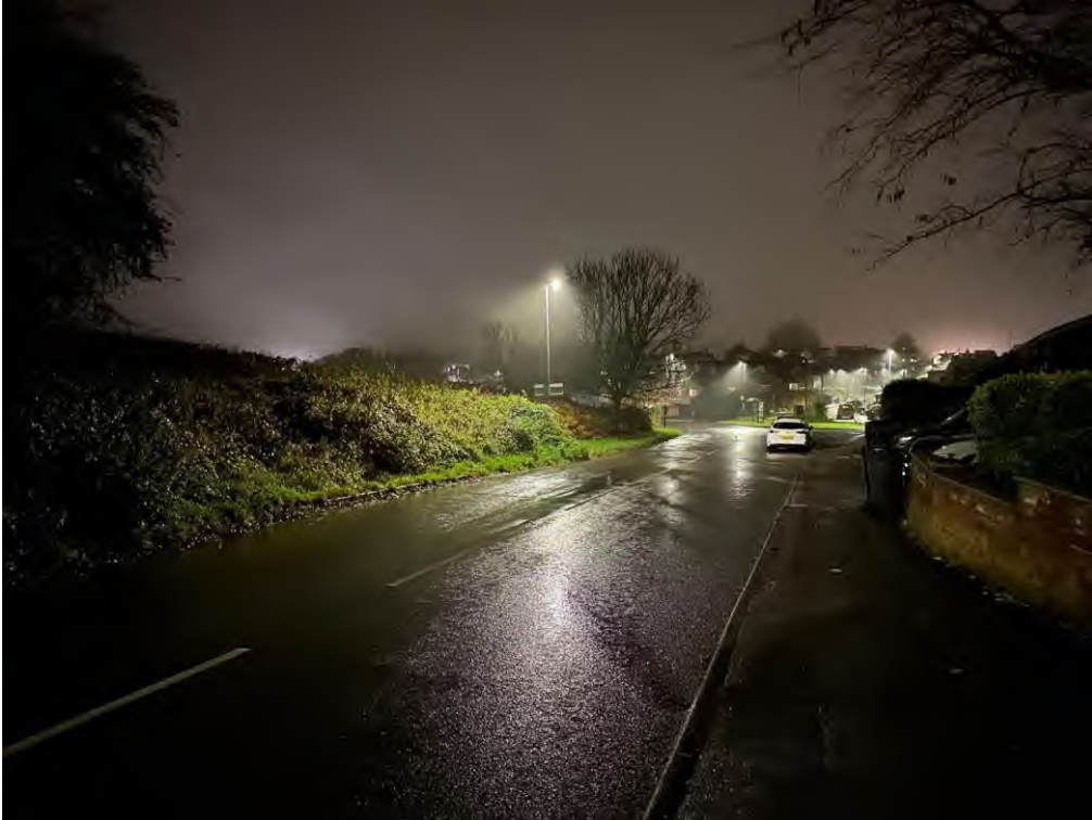
6.1 General view looking southeast on Carisbrook Road towards the proposed junction.
