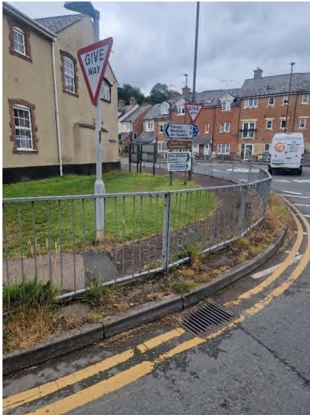
Image 7.6: Cluttered Street Signage at Abenhall Road/A4136 Junction - Visibility Left
