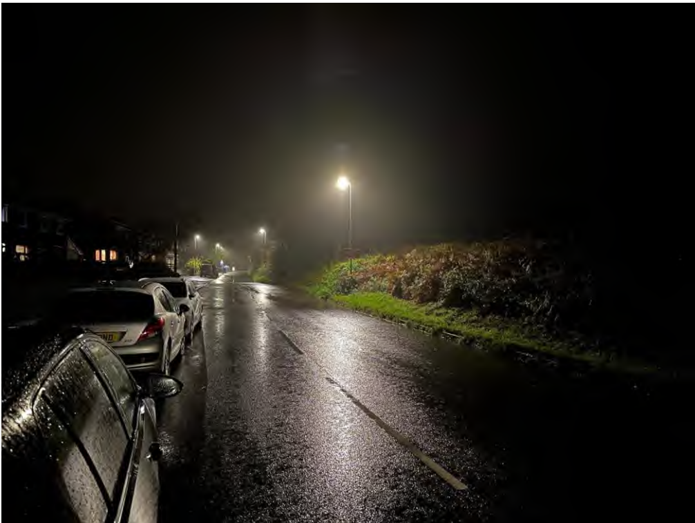
6.2 General view looking northwest on Carisbrook Road towards the proposed junction.
