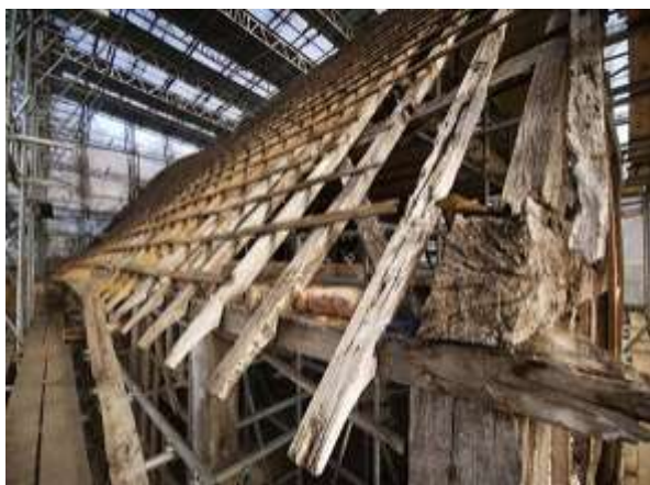
The roof has been stripped back to allow a detailed survey to be done, The pictures show just how frail the building is.
