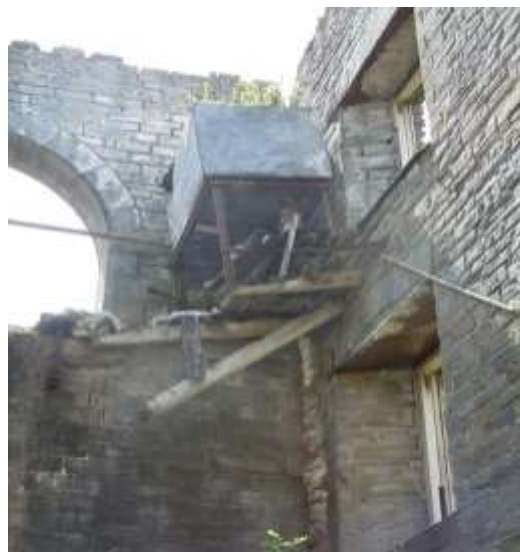
2017 the Pumphouse is only a shell, all the floors are gone, roof structure and the masonry is very loose in various areas. This building is at high risk of collapse.
