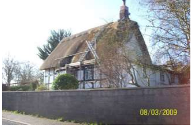
Undergoing rethatching of the roof 2009
