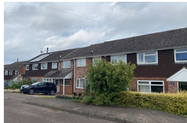
Figure 47: Typical hedgerow boundary.
