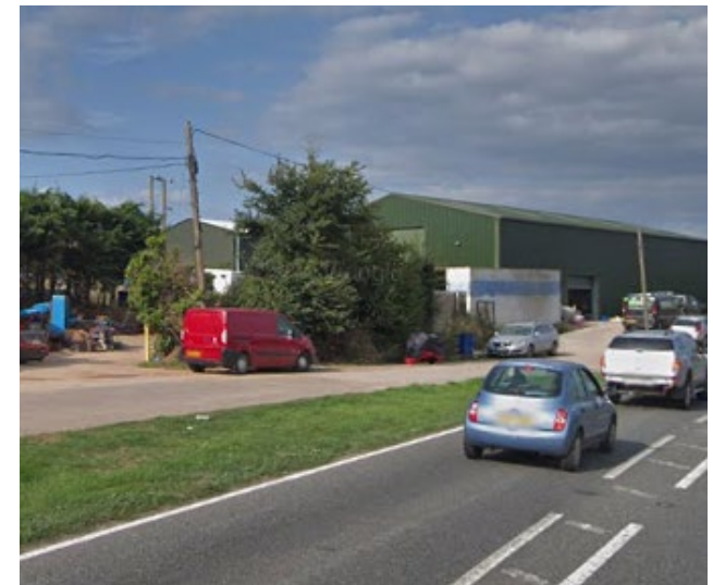
Figure 37: Preston Cross commercial units.
