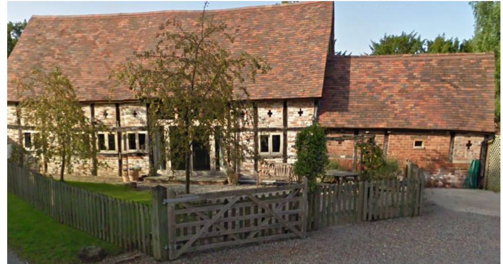
Figure 54: Where possible building materials or existing structures should be re-purposed with sustainability in mind. This image of an old barn converted into a residential dwelling is a good example of building re-use.
