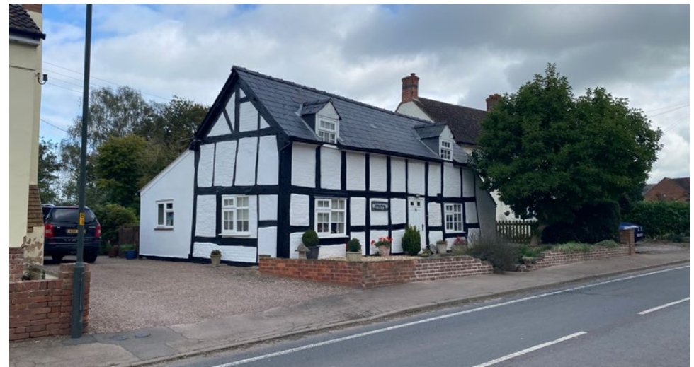
Figure 42: Typically buildings are residential, detached houses of two storeys or bungalows.
