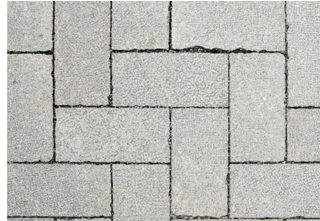
Figure 56: Permeable paving laid onto open graded bedding, base and sub-base layers allow percolation of water into earth.
