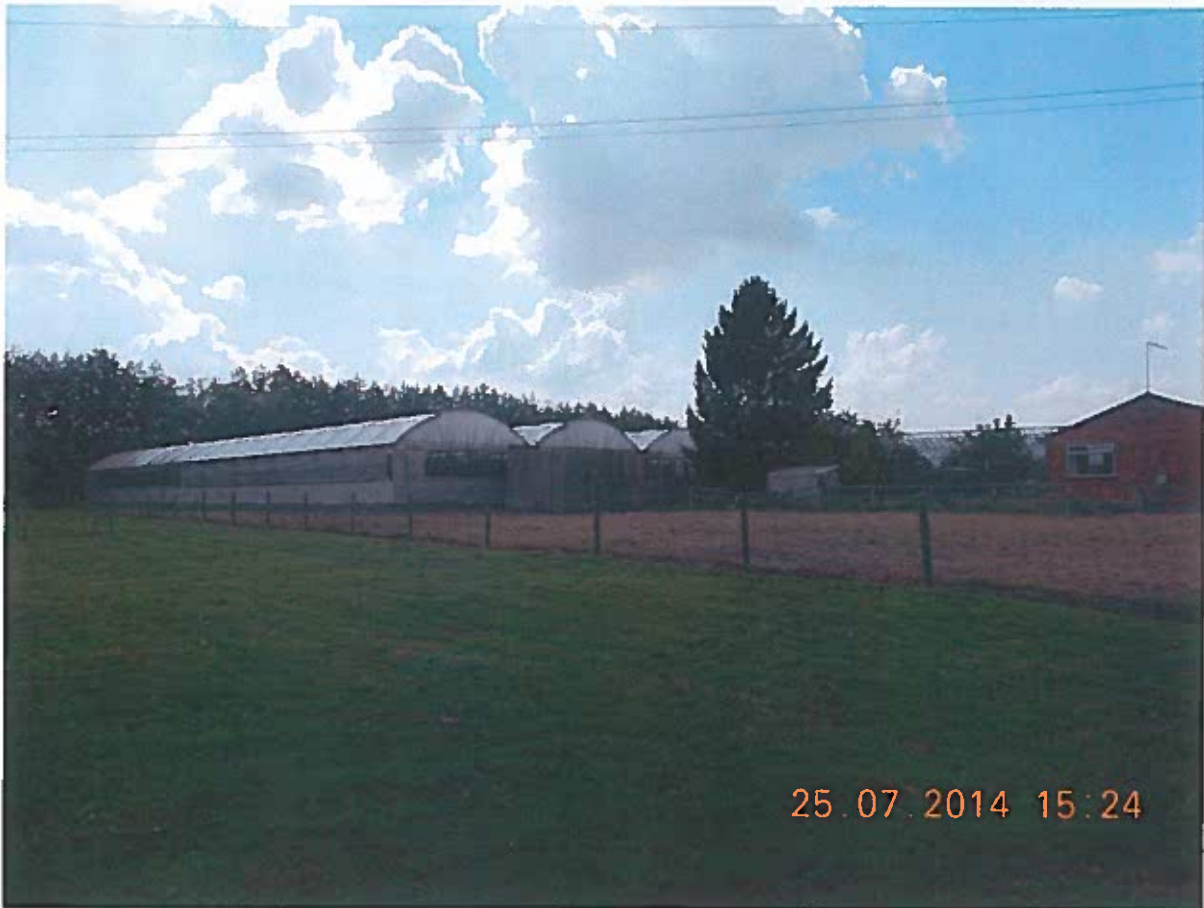
Above: Case Officer photo. A1 seen behind existing glasshouses viewed from Southend Lane
