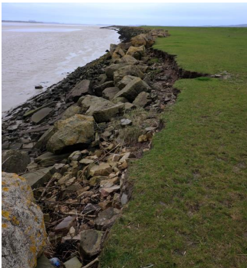
Photographs 1 & 2 – Sea wall erosion near Lydney
